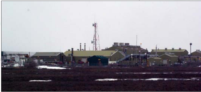
File photo of Pump Station 3, taken in Spring 2009—Mark Morones, JPO/SPCO
